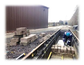
so this has been extended by the length of the new building. Construction of this structure required the use of over 750 concrete blocks and about 20 tons of concrete. The turnout into the service road from the yard has also been lifted to ensure that the track in the new shed will be level.
